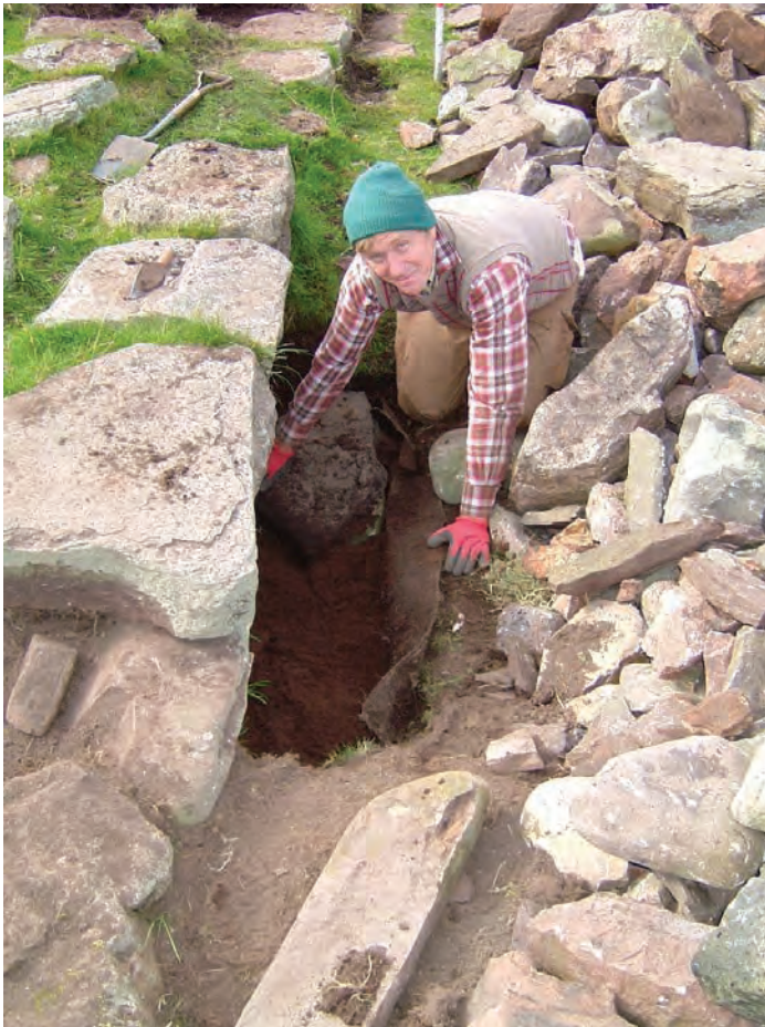
Fig. 7. Espen Martinssen underpinning the original foundations of the vernemur
